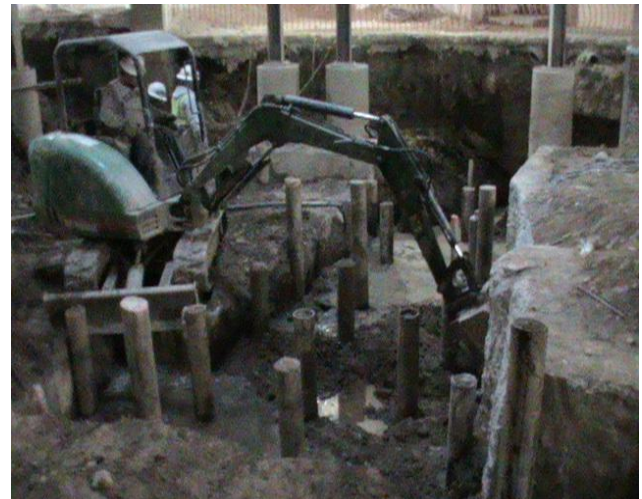
Figure 5 the photos above show the extent of the Micro pile installation and help convey the challenge of installing a new structural system below an existing building
