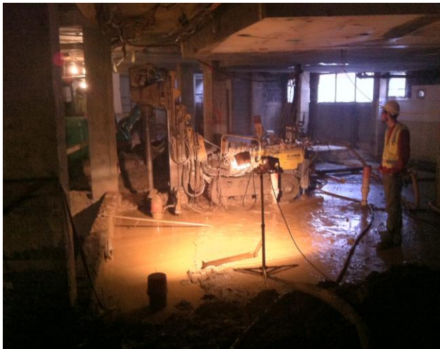
Figure 5 the photos above show the extent of the Micro pile installation and help convey the challenge of installing a new structural system below an existing building
